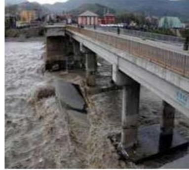
**Picture 7.** A collapsed bridge flood
